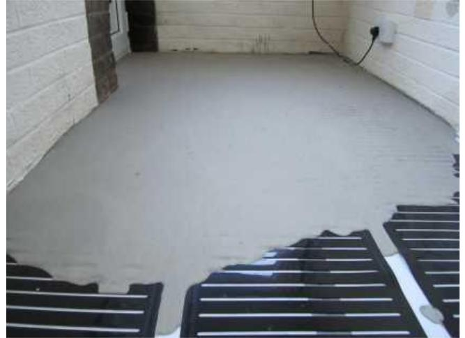
Wiring up matting elements and then covering with a self-levelling compound
