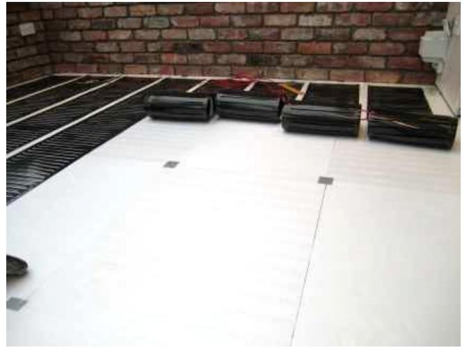
Laying out matting elements on top of Kapron Insulation board.
